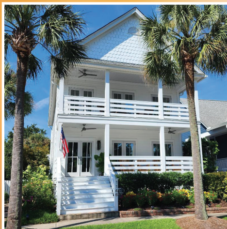
1146 Barfield Street, Alison and Casey Kellermann
